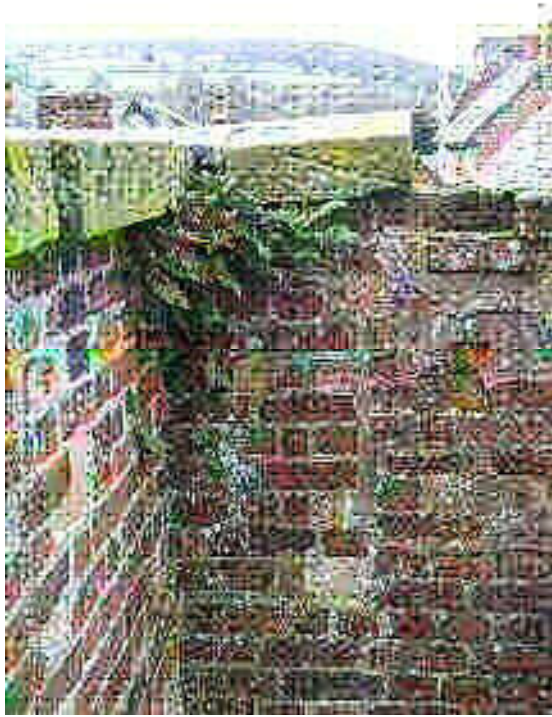
Fig 7: Detail to show plant growth and hard mortar pointing
