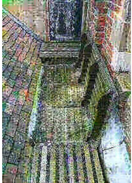
Fig 4: Detail to show the duck boards
