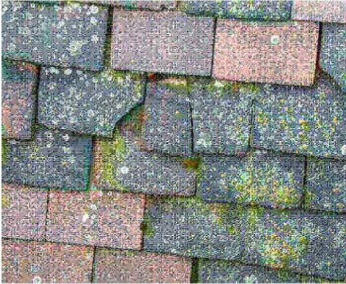
Fig 3: Detail to show damaged tiles
