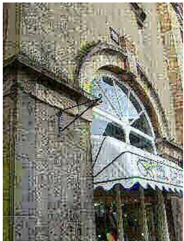
Fig 13: Detail to show inappropriate bracket fixed to building
