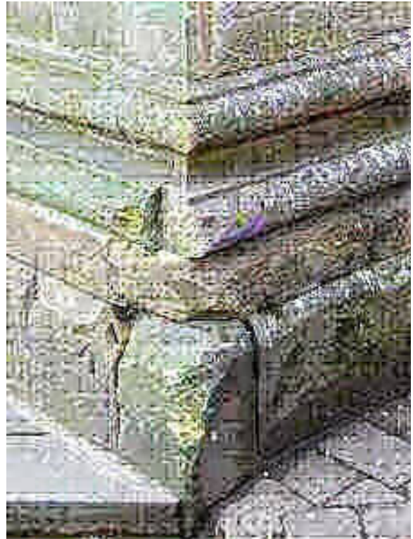
Fig 11: Detail to show low level vehicle impact damage to building
