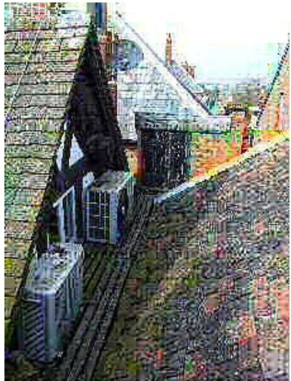
Fig 6: Detail to show air conditioning units fixed to duck boards
