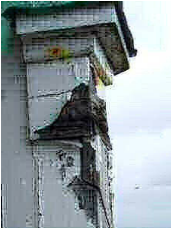
Fig 16: Detail to show wet rot decay to cupola post
