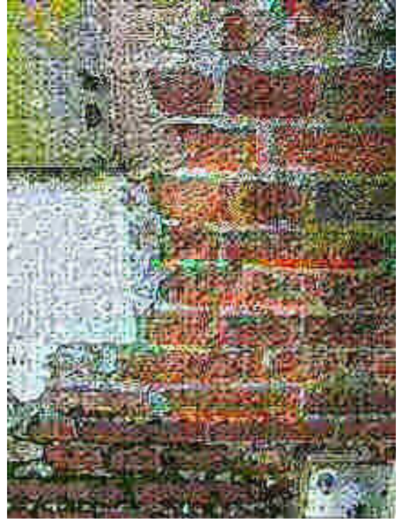
Fig 8: Detail to show spalled brickwork
