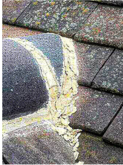
Figure 1. Spalled mortar bedding of ridge tiles.
